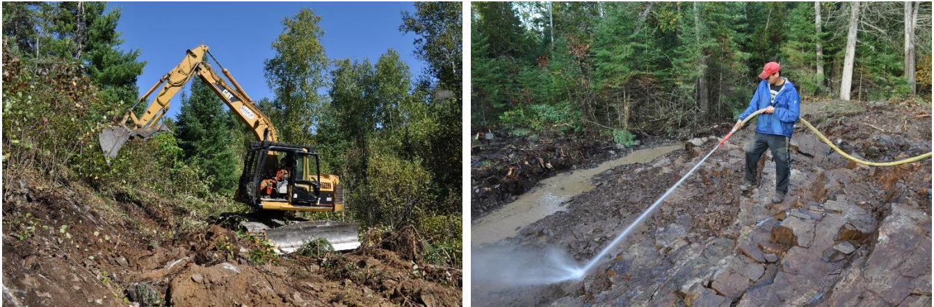
Stripping high priority, near mine, targets (left – removing overburden; right – washing down prior to mapping and sampling)
