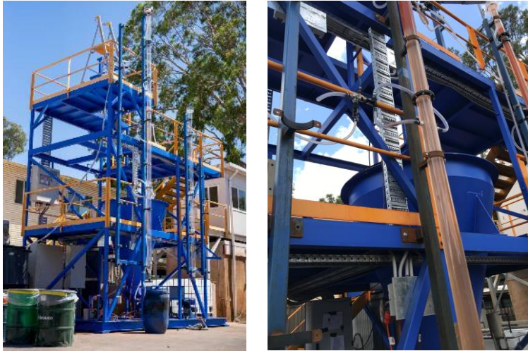
1. SALT PILOT PLANT (UNDER CONSTRUCTION)
