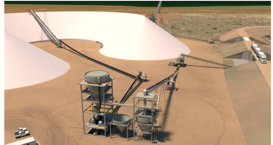
2. SALT WASH PLANT
