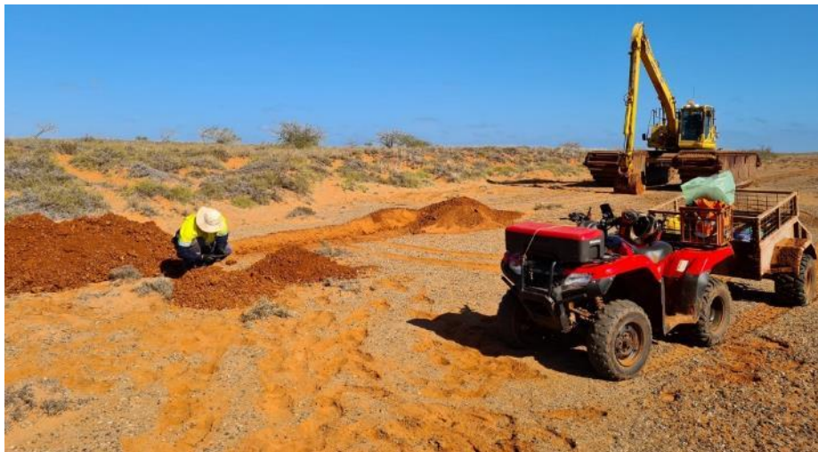
3. GEOTECHNICAL TEST PIT FOR FEED
