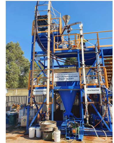
SALT PILOT PLANT (PERTH)
