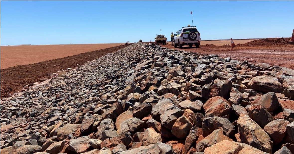
Figure 3: Northern Embankment Trial – Rock Armoured Wall
