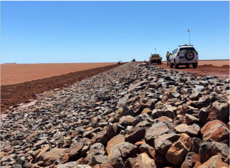
NORTHERN EMBANKMENT TRIAL
