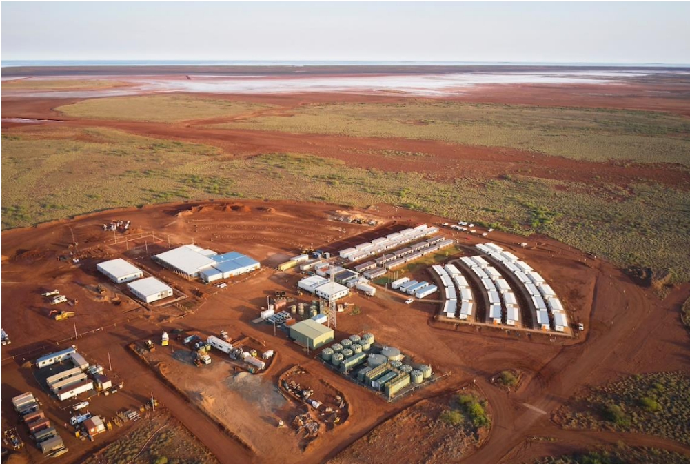
Construction progress from 200 to 400 beds
