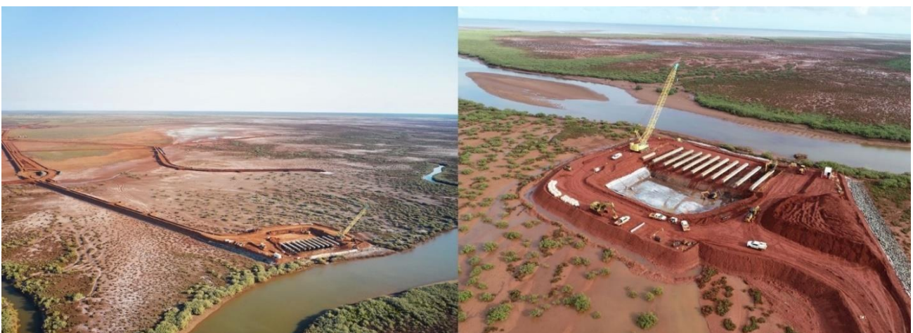
(L) Access levee to seawater structure; (R) Construction of seawater structure
