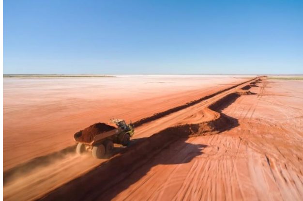
Figure 2: Pond 1 levee construction
