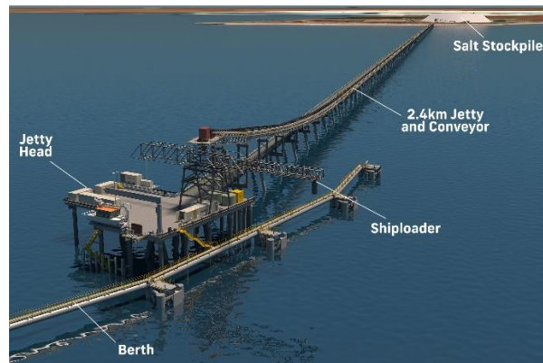
Figure 5: Jetty on completion
