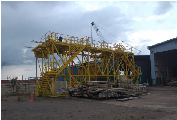
Figure 4: Jetty traveller construction
