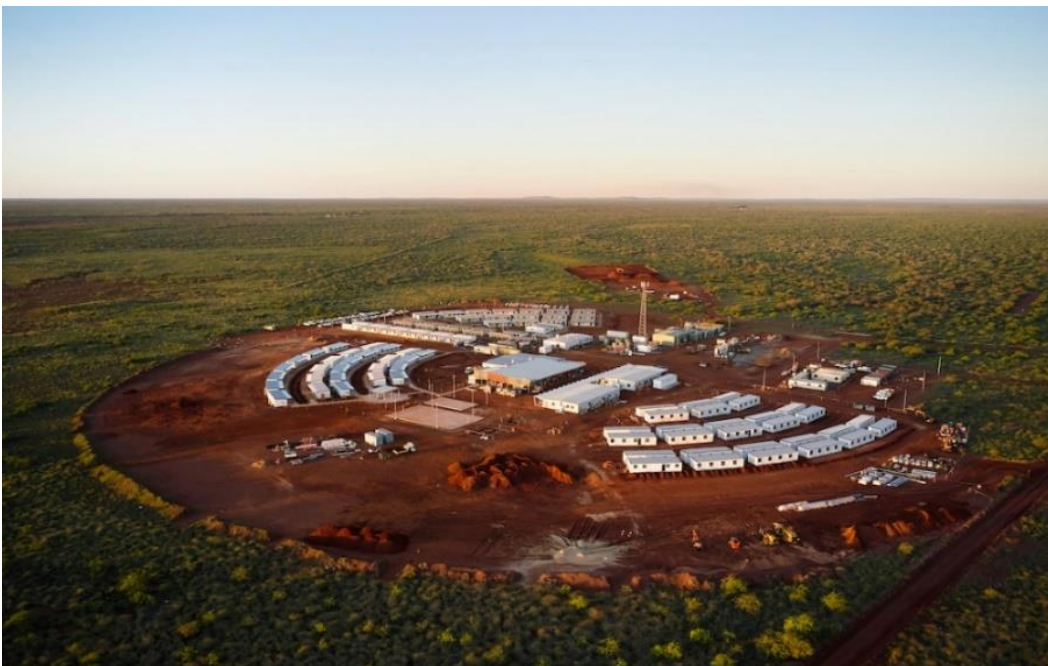
Figure 3: Accommodation Village construction
