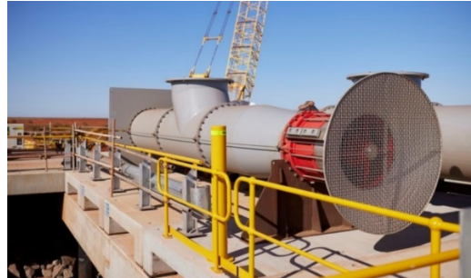
Figure 2: Intake Pump Installation
