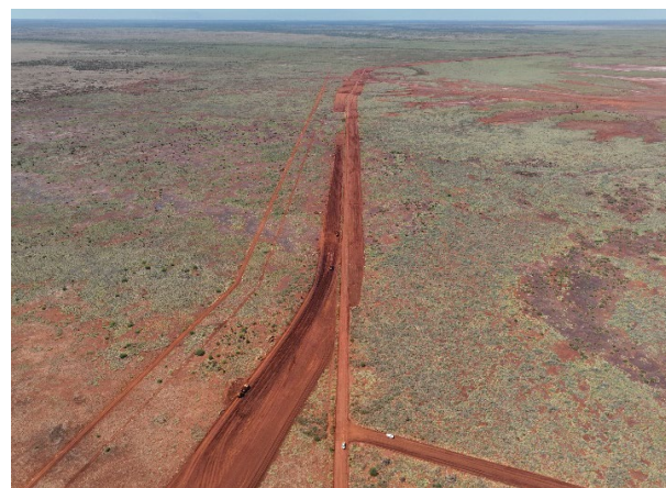
Figure 7: Works continue on the North South Road
