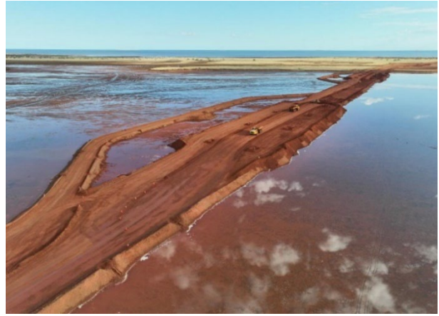
Figure 2: Causeway culvert infills
