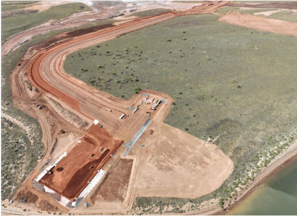
Figure 1: Construction commenced on causeway and jetty laydown area
