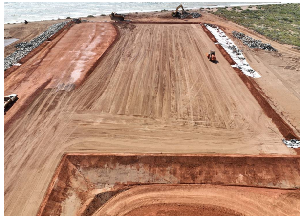
Figure 4: Assembly pad at jetty island
