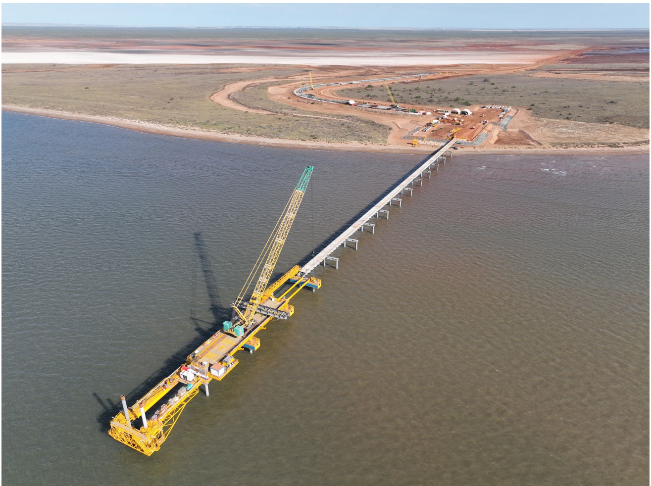
Image 1: 2.4km Marine Structure Progress
