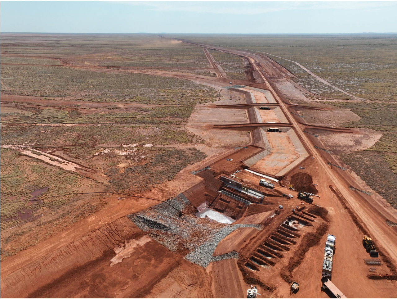
Image 4: Civil works at Transfer Station between Evaporation Ponds 2 and 3
