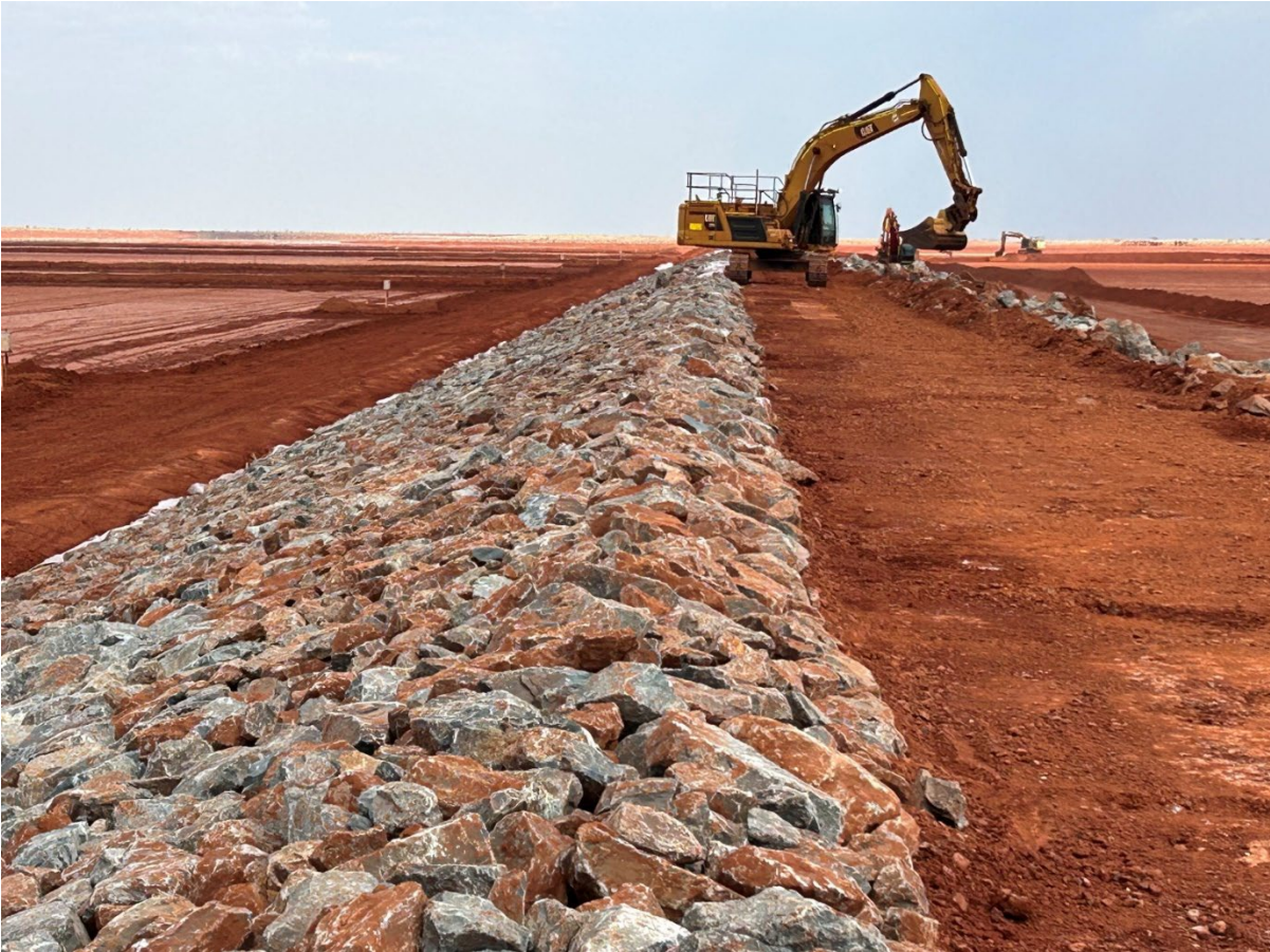
Image 2: Rock embankment to strengthen pond walls
