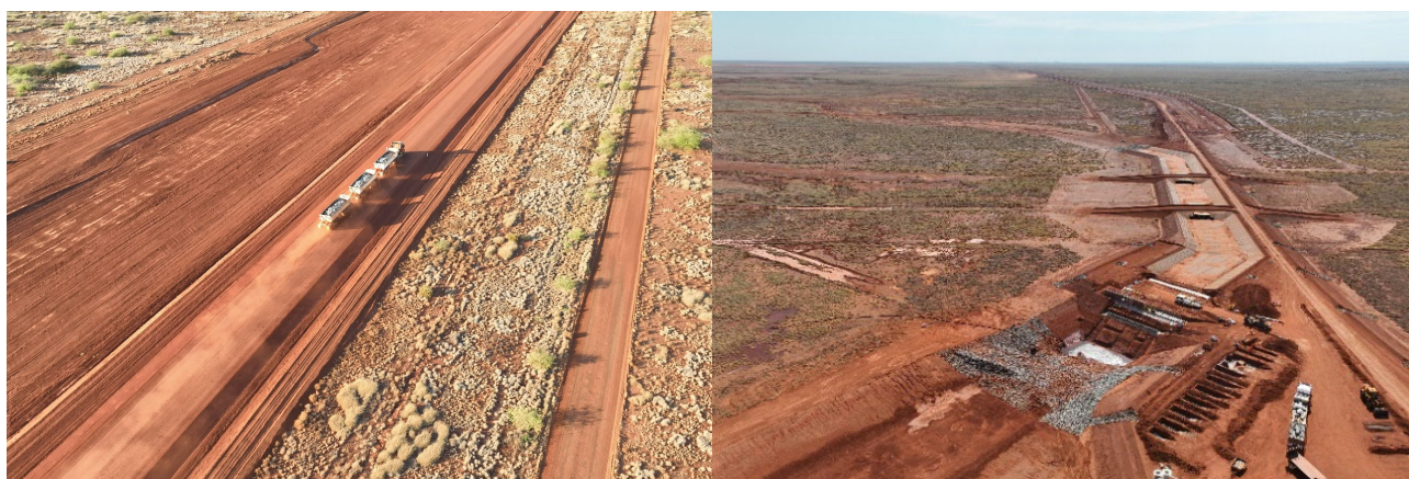
Image 1: Rock delivery on completed Mardie Road
