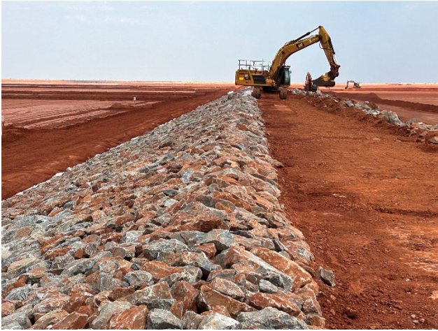
Image 3: Rock embankment construction
