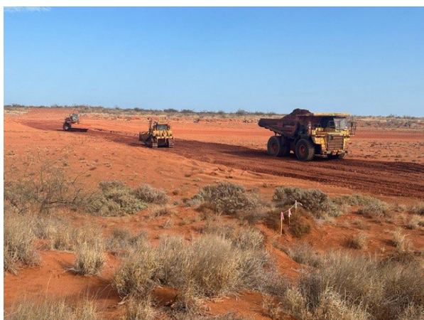
Figure 3: Pond 6 access road
