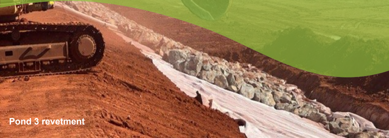
Pond 3 rock armour placement
