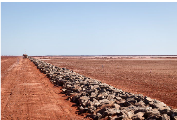
Figure 4: Evaporation pond rock wall
