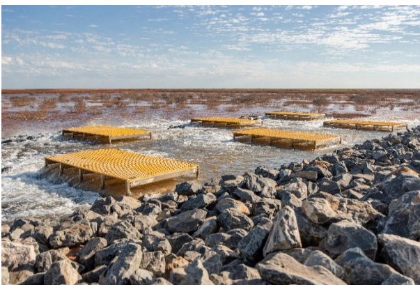
Figure 1: Seawater flowing through the Primary Seawater Intake Station
