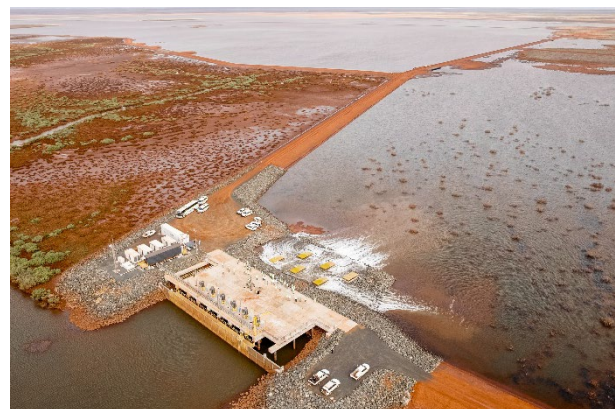
Figure 2: Seawater flowing into Pond 0
