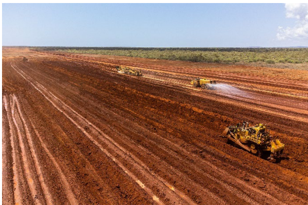
Figure 3: Construction of the crystallisers within the OMP area
