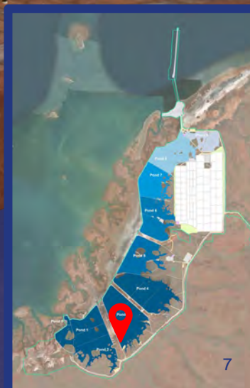
Commissioning of transfer station 2/3
