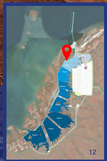
Rock armour on pond 8 seawall
