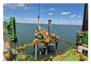
Figure 4: First jetty head piles installed
