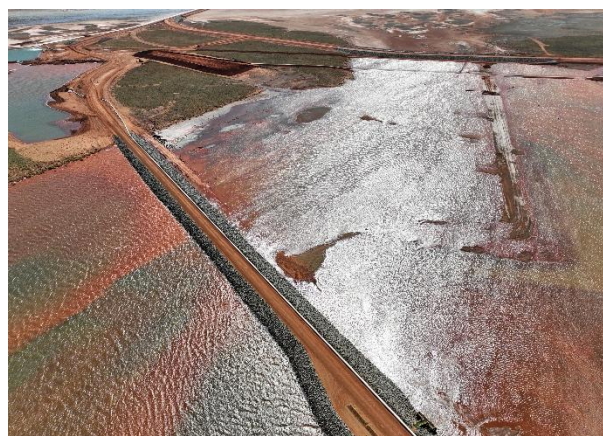
Figure 2: Water inundation at pond 9
