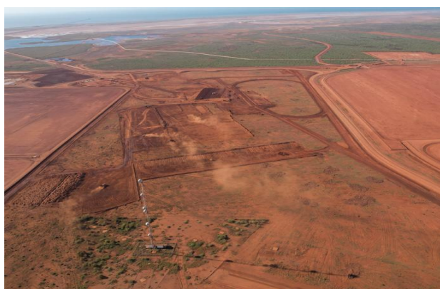
Figure 3: Salt wash plant earthworks commencing
