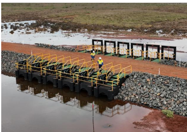
Figure 1: Culvert between pond 7 and pond 8
