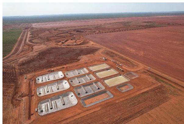
Figure 6: SOP Pilot Ponds being constructed and commissioned
