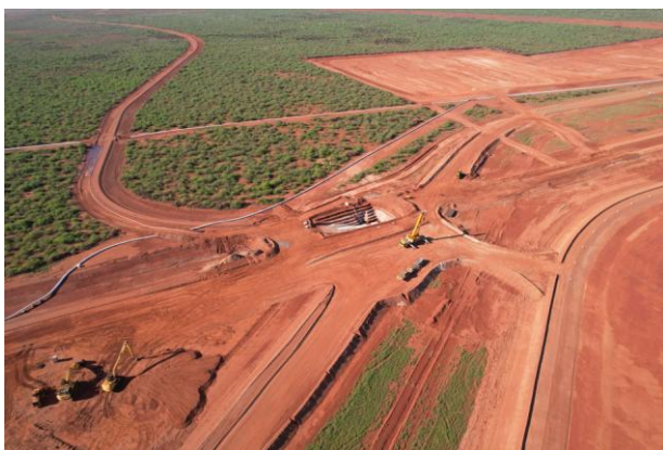
Figure 5: Lift station under construction
