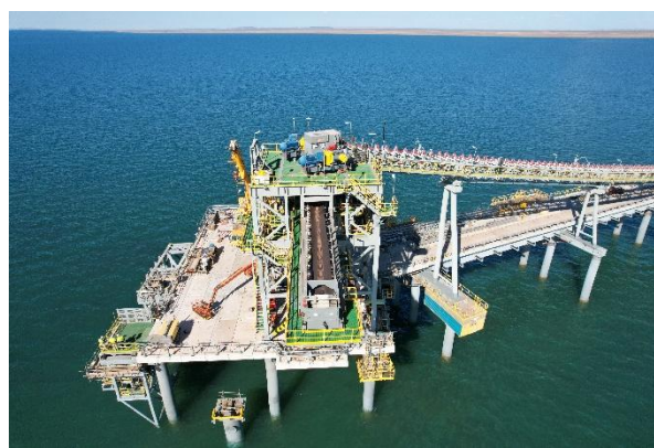
Figure 4: Jetty Head Works nearing completion
