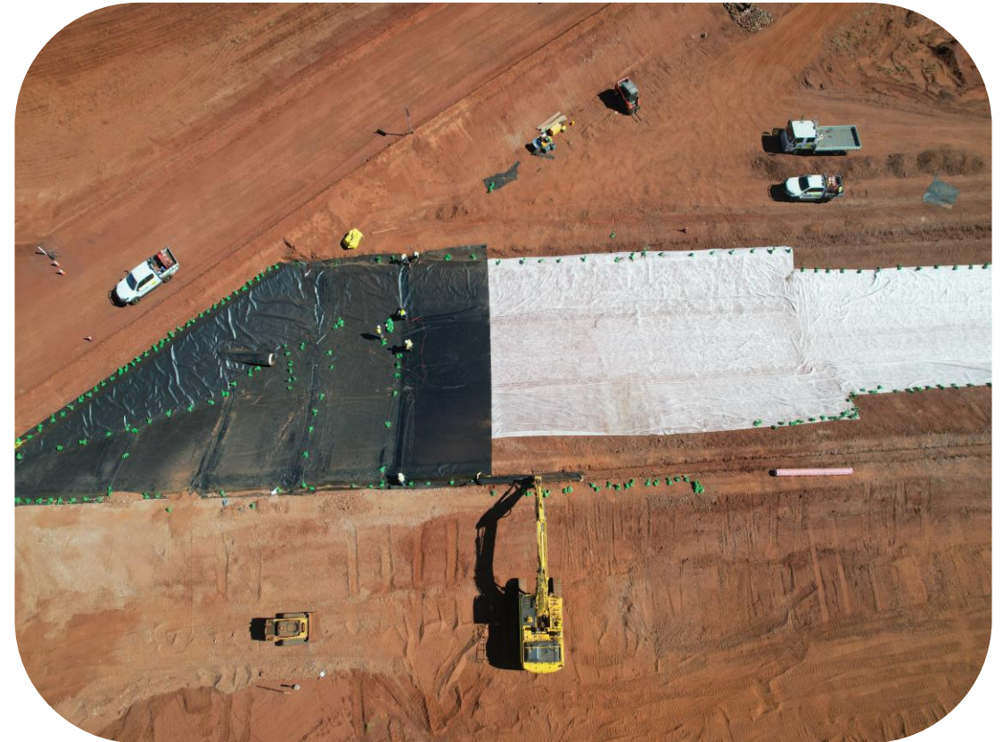
Brine channel liner installation
