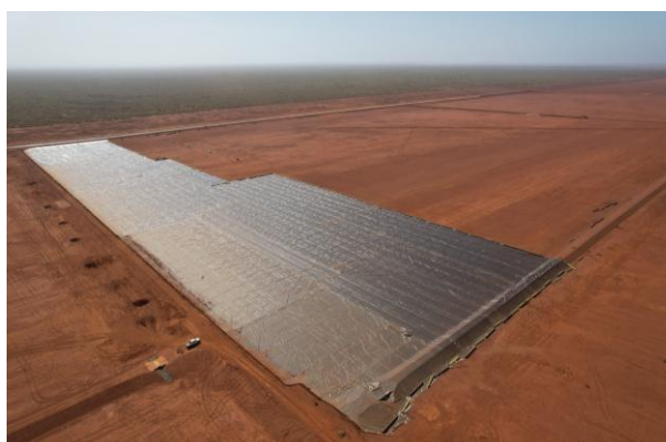
Figure 4: Crystalliser pond lining
