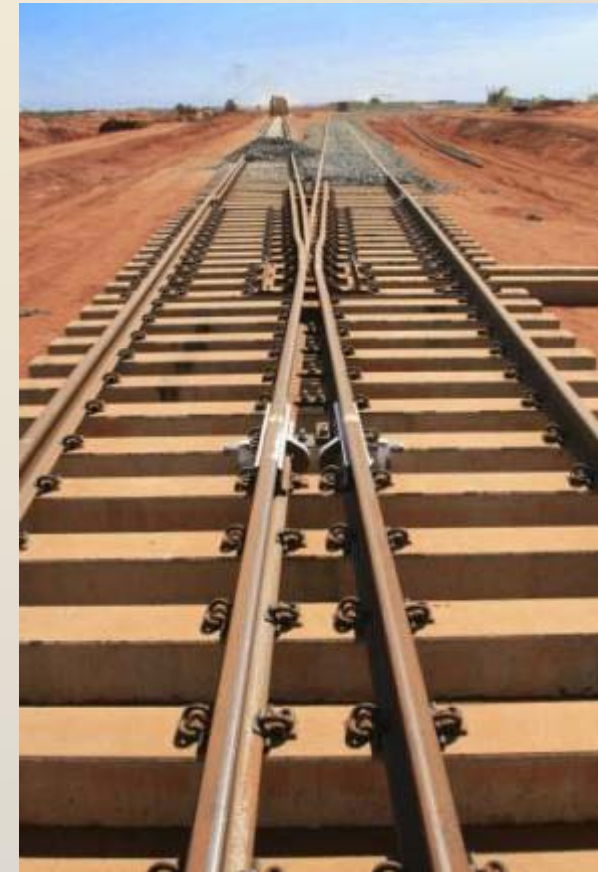
Fortescue track laying ( www.fmg.com.au )
