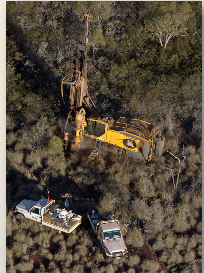
Drilling at Coongan Well
