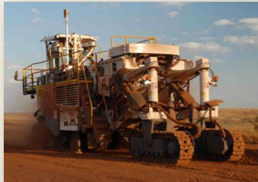
Wirtgen 2500SM commences at Outcamp Well - NIOJV
