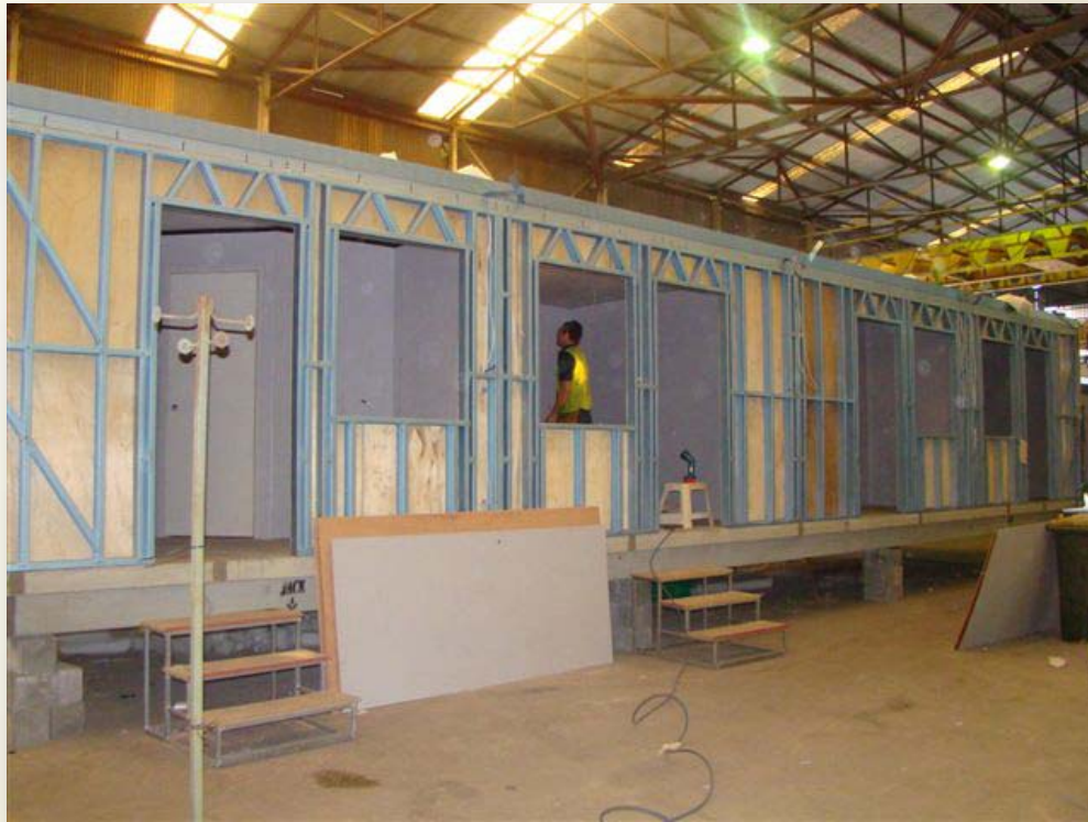
Phase 1 camp units under construction
