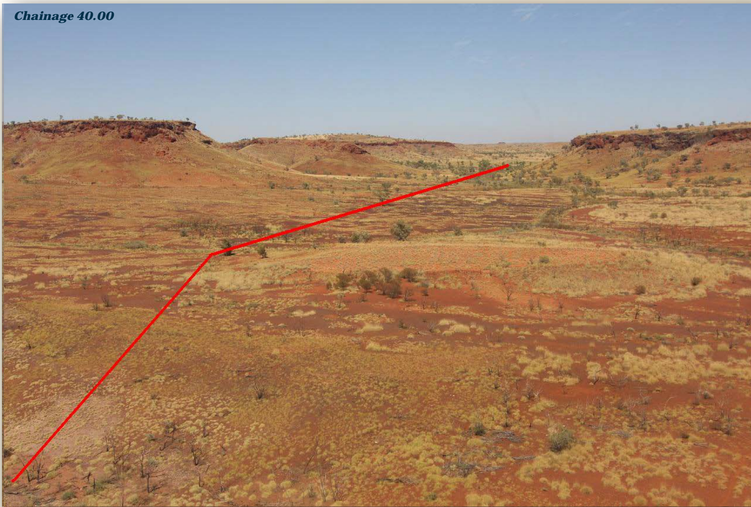
Haul road route aerial survey
