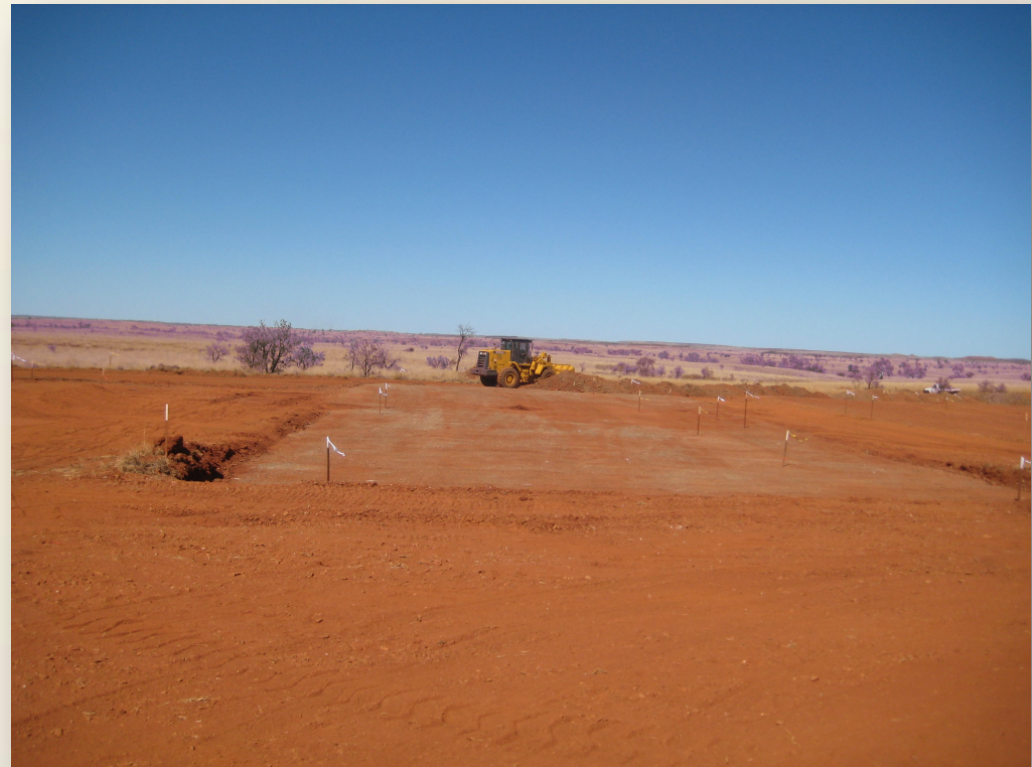
Phase 1 camp under construction
