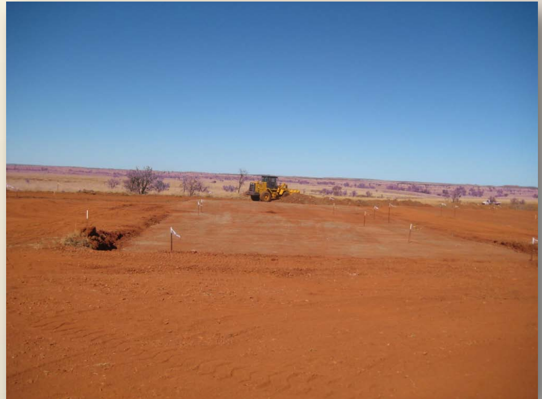
Phase 1 camp under construction
