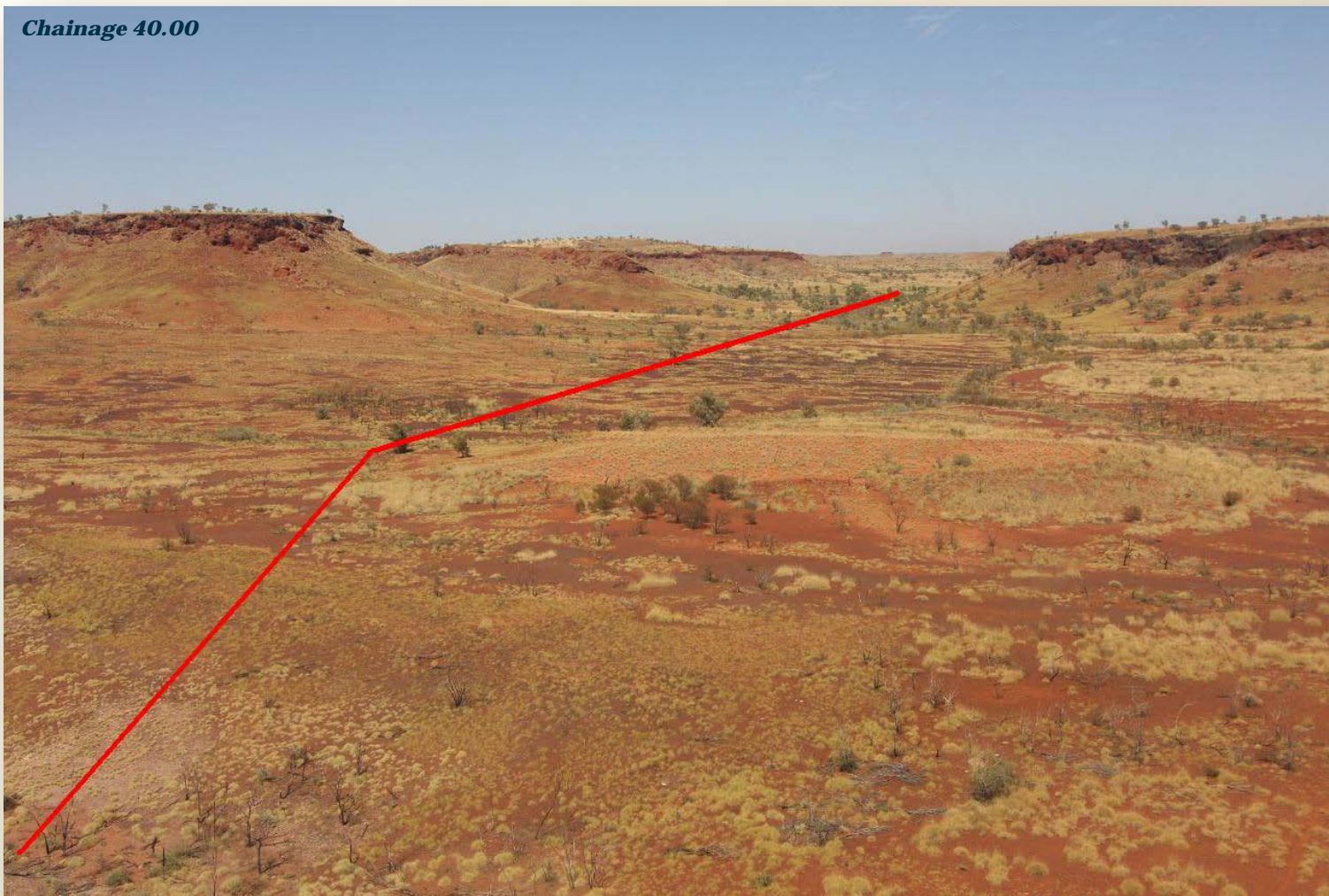
Haul road route aerial survey – Chainage 40.0 – view south
