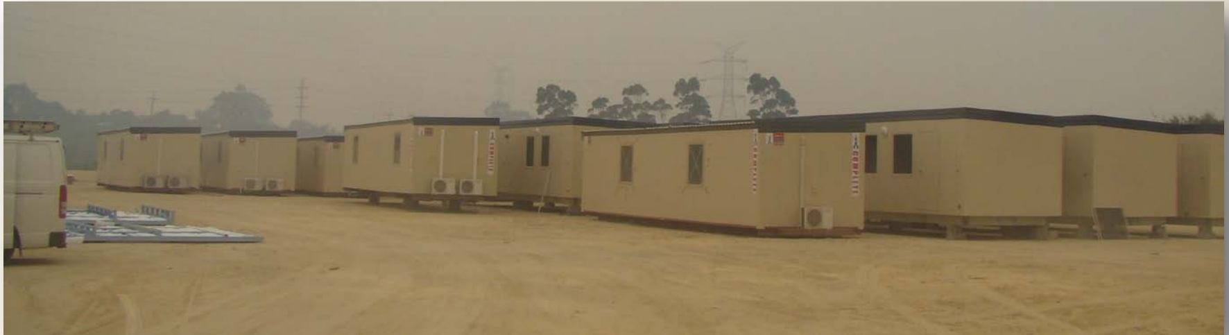
Complete Portables - Phase 1 camp units being prepared for transport
