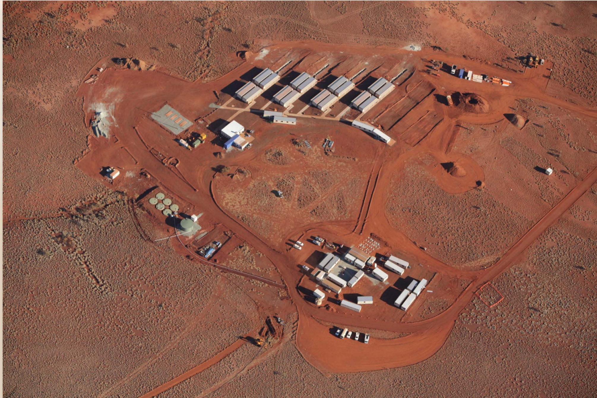
Aerial view of BC Iron first stage, 60-man camp. Expansion underway to final camp which will be 180-man.
