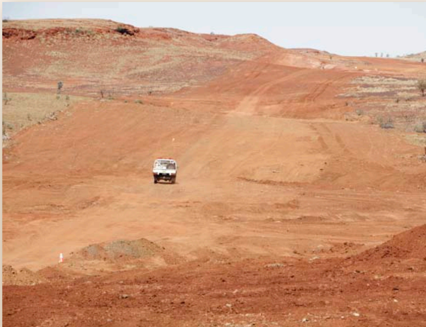
Haul road alignment clearing (above).
