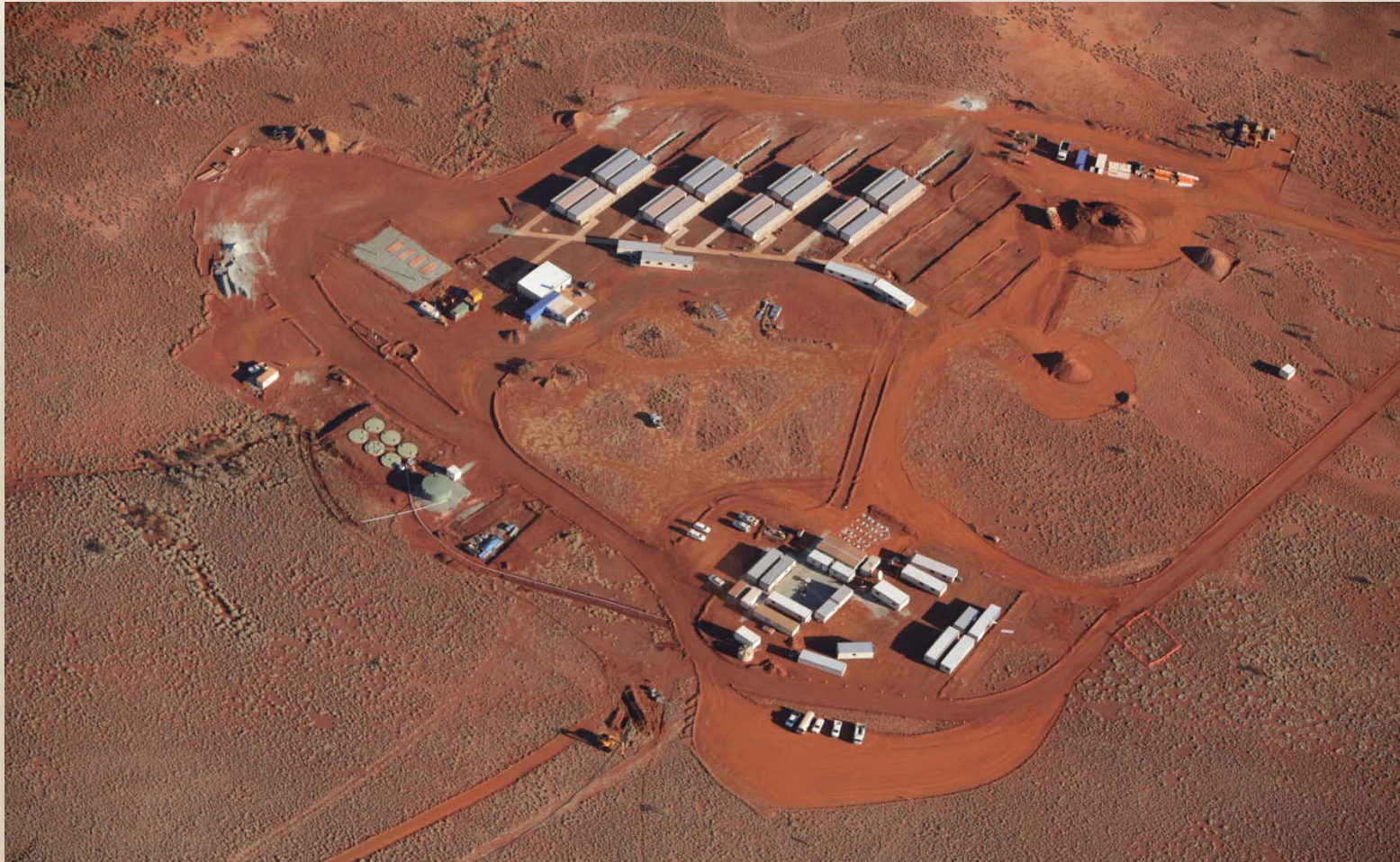
Aerial view of BC Iron first stage, 60-man camp. Expansion underway to final camp which will be 180-man.
