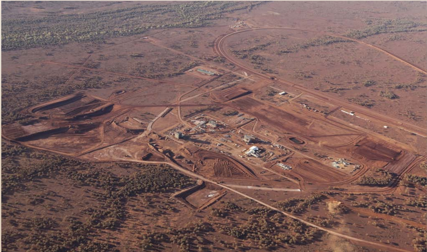
Aerial view looking southeast of Christmas Creek OPF rail loop. BC Iron stockyard area will be in the cleared area in the middle right of the photo.
