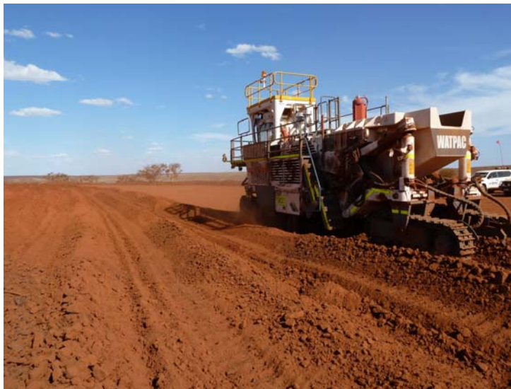
Image 1: Surface Miner in operation at Outcamp
