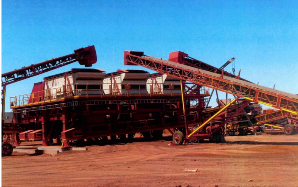
Image 2: Striker crushing & screening plant under construction at site
