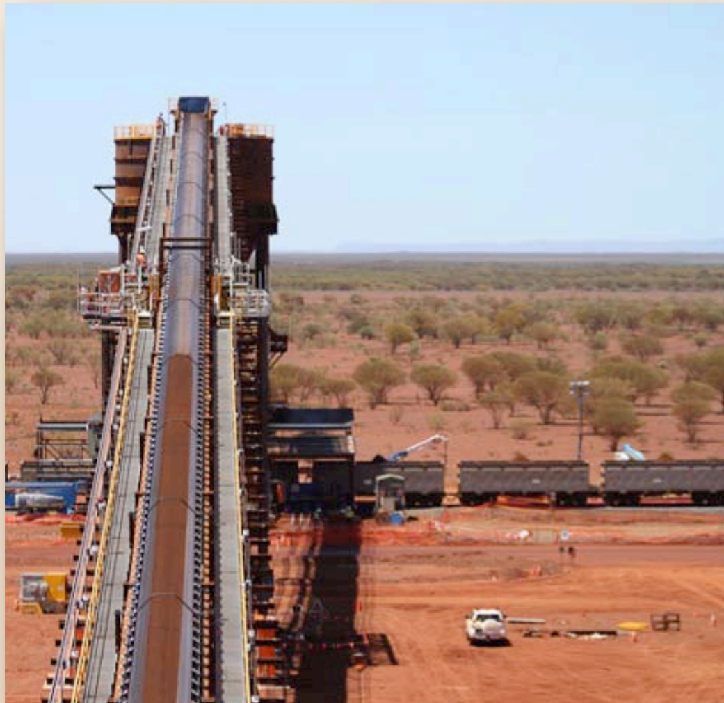
Christmas Creek train loader loads BC Iron's first train, Feb 2011
