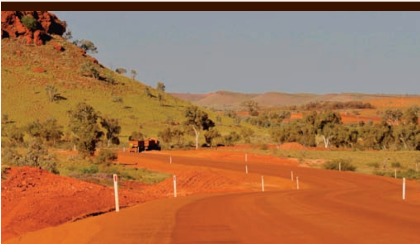
Private Haul Road Through the Chichester Range
