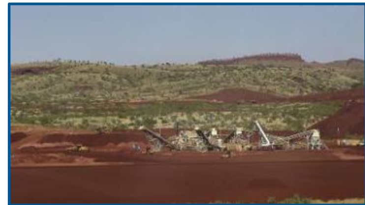
Iron Valley Commissioning – August 2014
