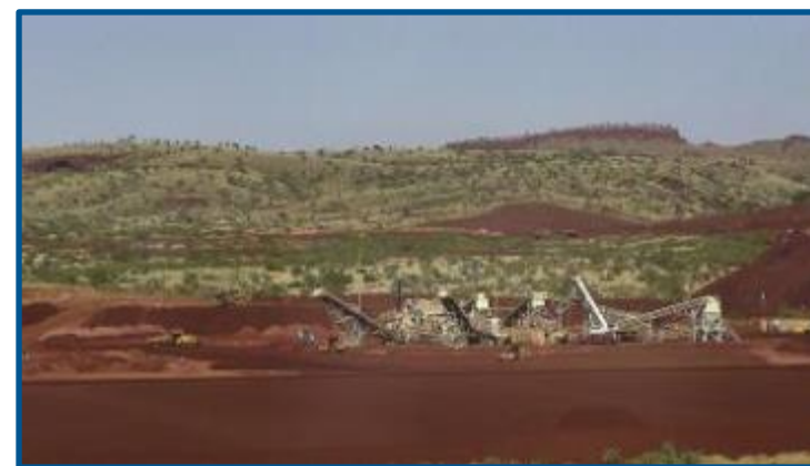
Iron Valley Commissioning – August 2014
