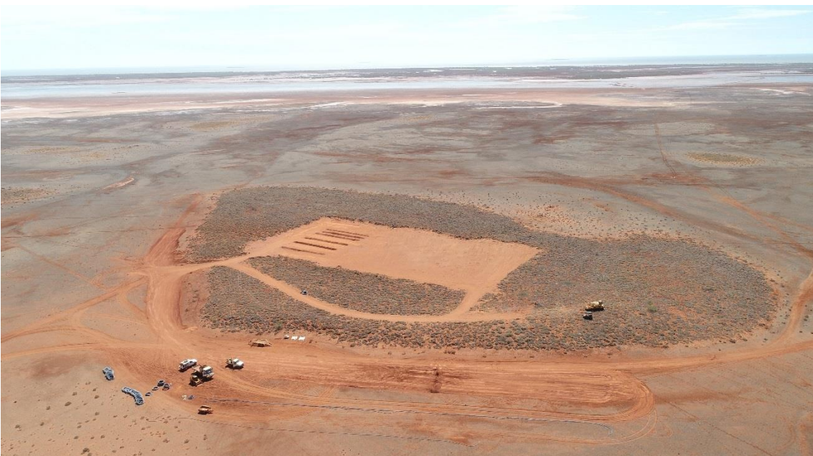
Figure 3: Small-scale Evaporation Trial Under Construction
