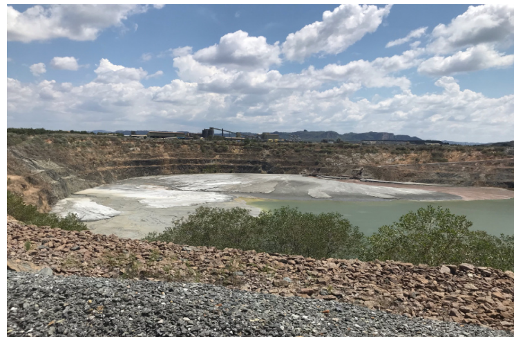
Pit 3 tailings deposition progress
