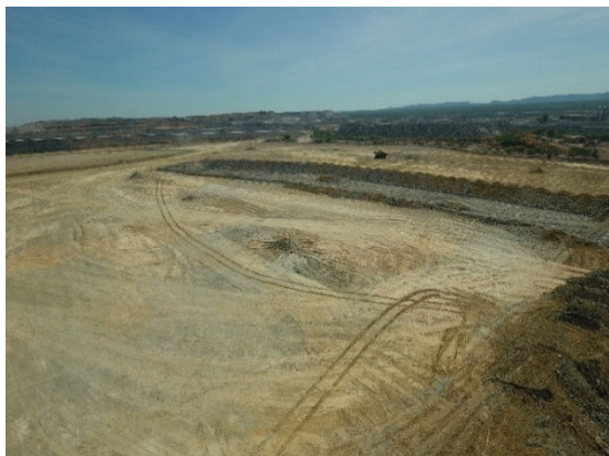
Pit 1 backfill - final stages
