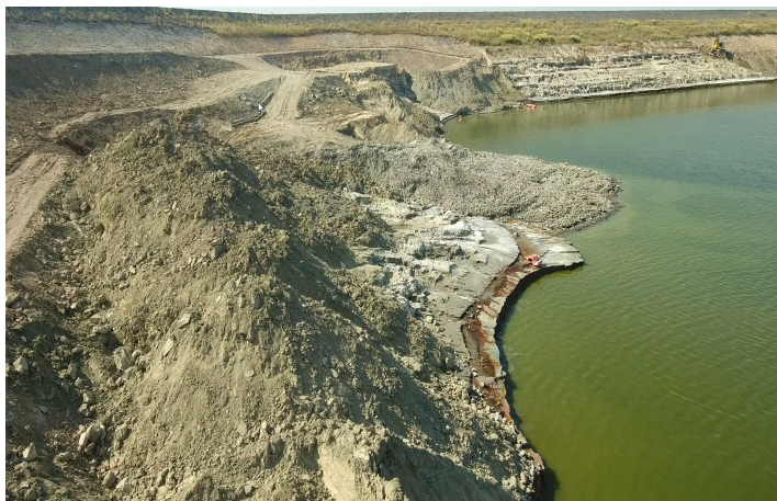
TSF Wall Cleaning
