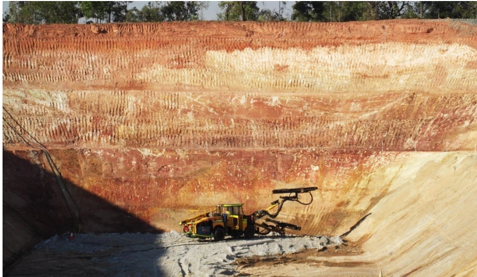
Ranger 3 Deeps exploration decline box cut 18 July 2012
