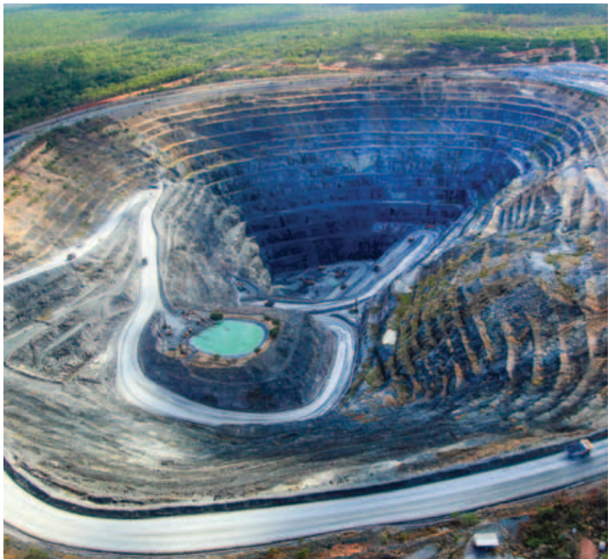
Open cut mining concluded after 31 years of operation. Backfilling of Pit 3 has now commenced as part of Ranger mine's progressive rehabilitation programme.
