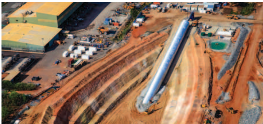
Ranger 3 Deeps exploration decline portal backfill underway in November 2012. The backfill of the box cut was completed in December 2012.
