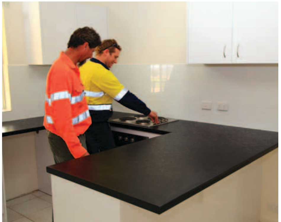
Trevor Beckman and Damien Reeves, part of the Infrastructure team who undertook upgrades to 60 ERA houses in Jabiru
