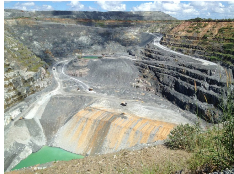
Over ten million tonnes of waste rock has been backfilled in Pit 3 at 23 April 2013
