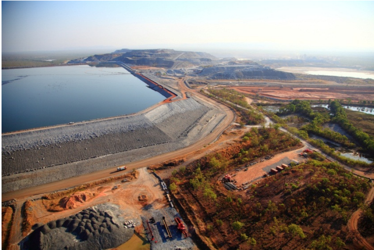
2.3 metres lift completed on the Tailings Storage Facility in 2012
