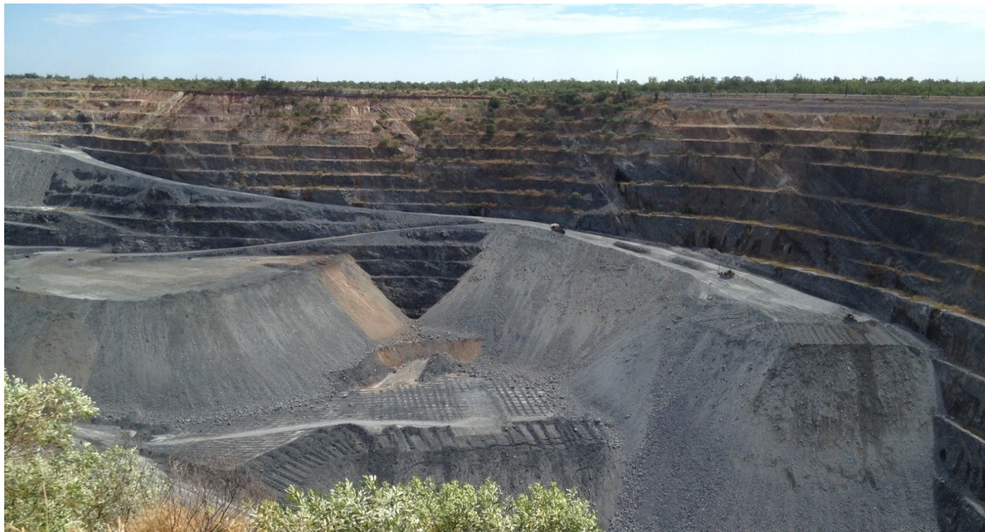
15 million tonnes of waste rock has been backfilled in Pit 3 as at 30 July
