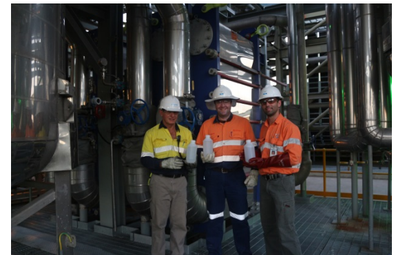
First distillate water produced
