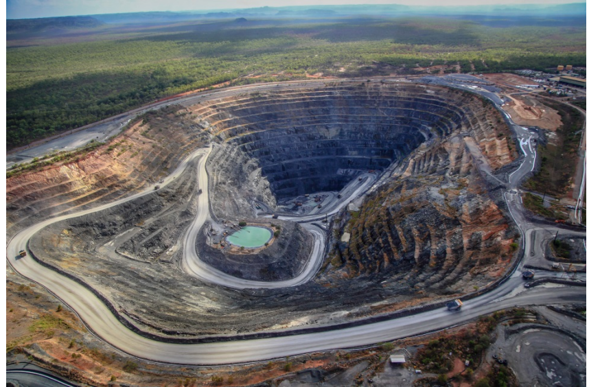
Pit 3 at completion of mining in November 2012
