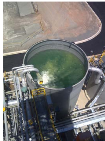
First process water introduced to Brine Concentrator
