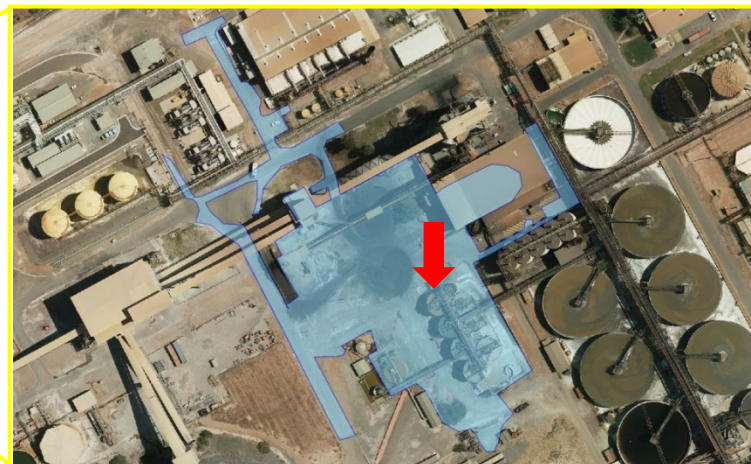
Leach Tank No. 1 (arrowed) and spill area
