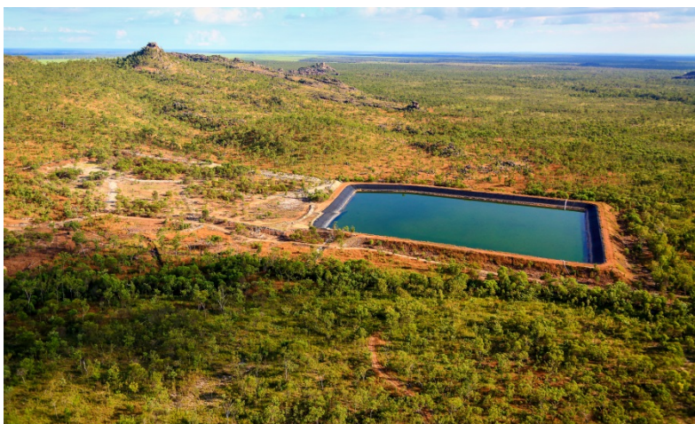
Jabiluka Interim Water Management Pond
