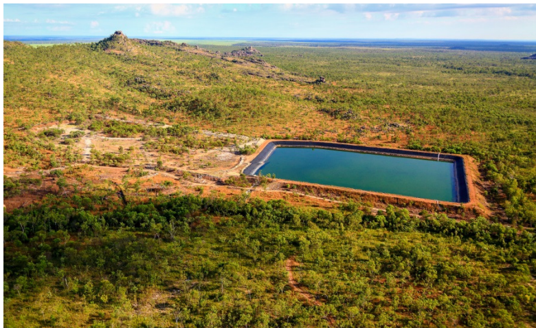
Jabiluka Interim Water Management Pond
