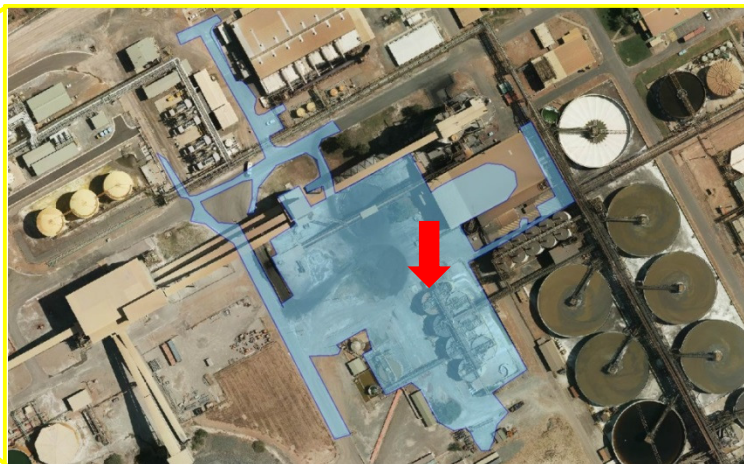
Leach Tank No. 1 (arrowed) and spill area
