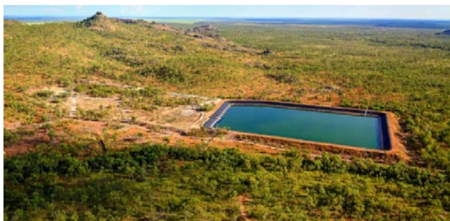
Jabiluka Interim Water Management Pond
