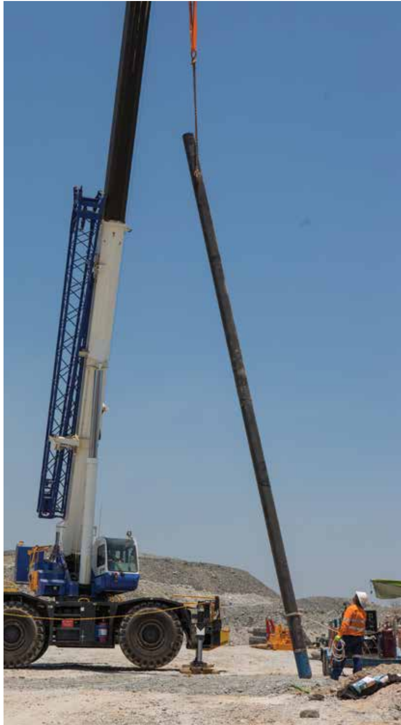
▲ Construction activities at Ranger
