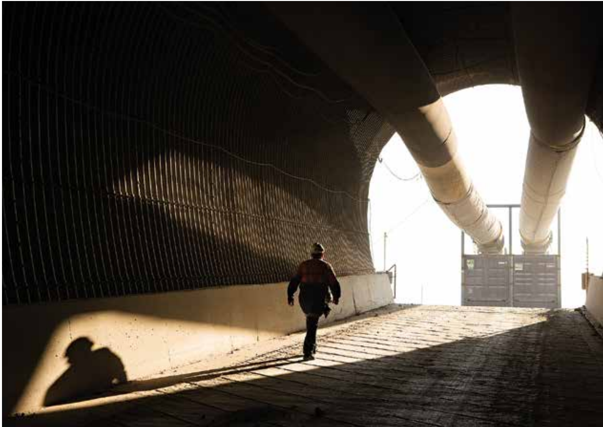
▲ The 185 metre long entrance portal for the Ranger 3 Deeps Exploration Decline
