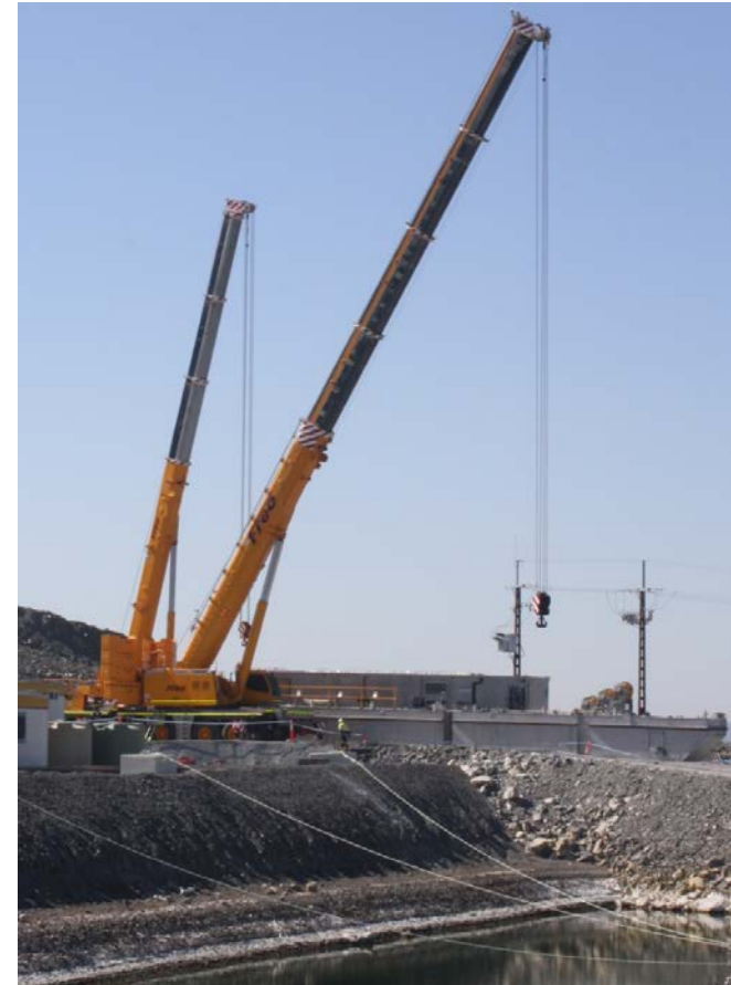
Construction of dredge at Ranger site in July 2015
