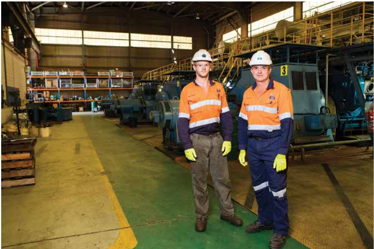
▲ Maintenance Trade Apprentice Dane Warhurst and Superintendent Darren Fairman in the Ranger Power Station
