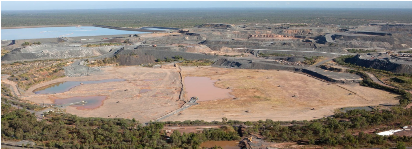
Laterite capping of Pit 1
