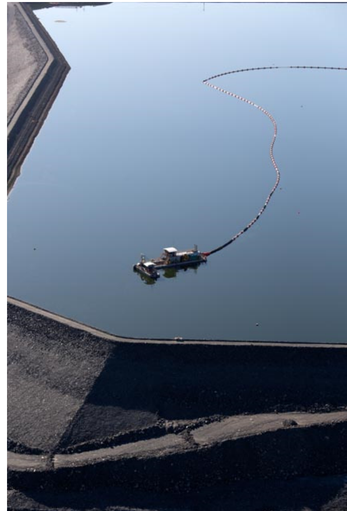
Dredging the Tailings Storage Facility
