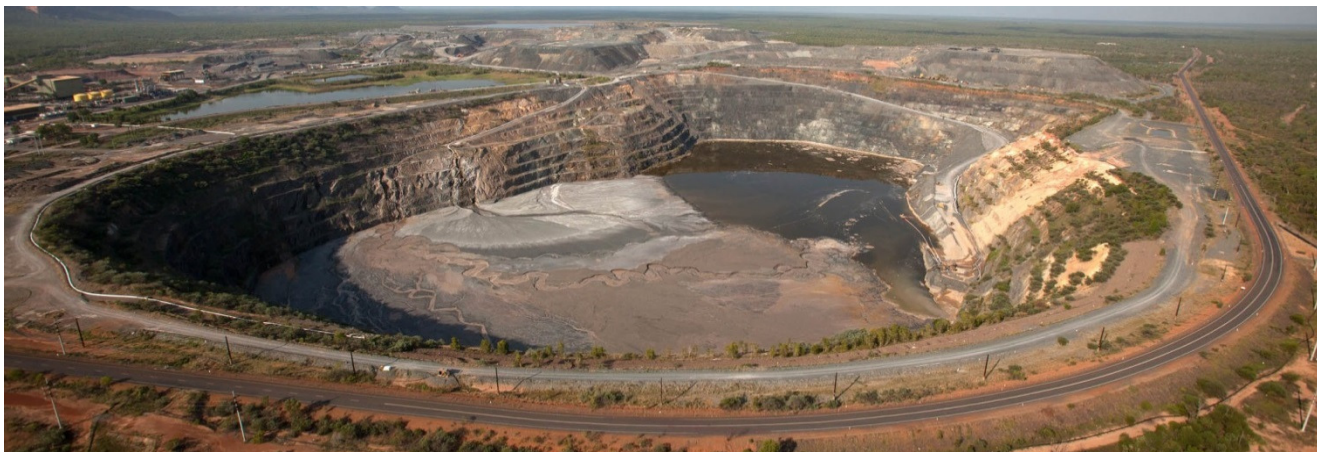
A tailings beach is forming in Pit 3 as part of the work to rehabilitate the pit
