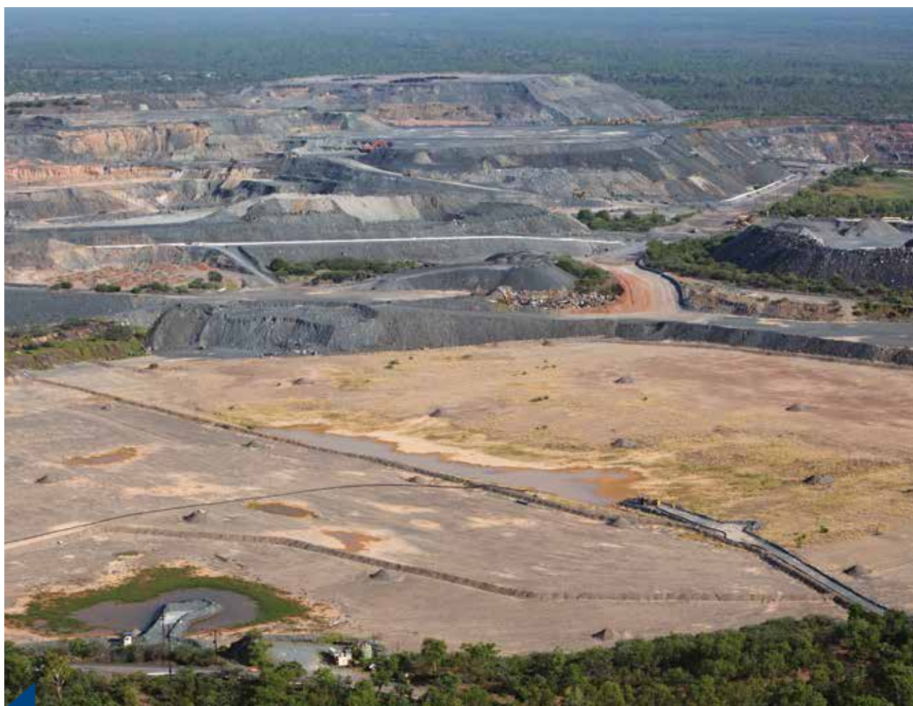
The capping of Pit 1 was completed in January 2016, the next stage of the rehabilitation process will be to commence bulk backfilling.
