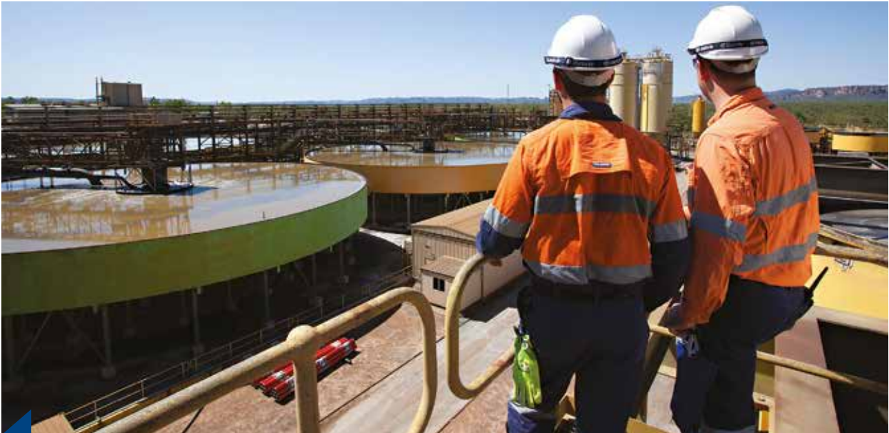
Engineers look over the processing area of Ranger mine.
